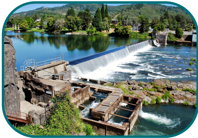
Winchester Dam and fish ladder on the North Umpqua River in Winchester, OR. Credit: EWY Media/Shutterstock
