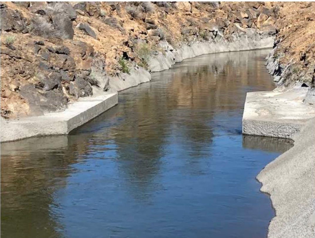
Flow Measuring Site within recently constructed reach
