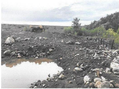
Above: Excavation and grading of upper end of site
