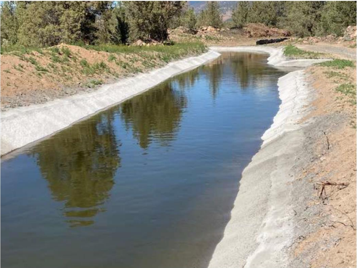
Looking downstream at canal lining reach completed in spring 2021.
