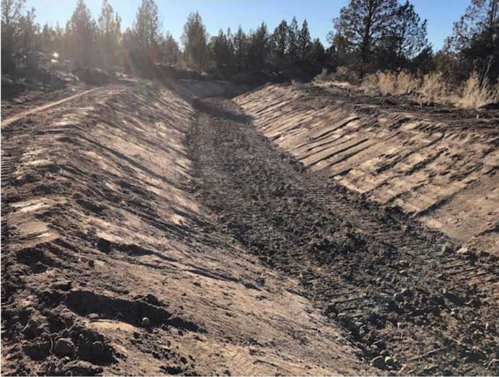
Canal reach being prepared to receive geo-membrane liner
