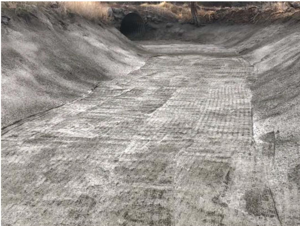
Main Canal lining at Hwy A-12 culvert crossing
