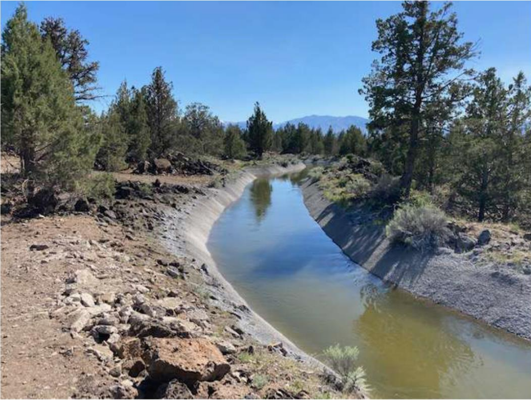
Reach of recently lined canal during spring of 2021
