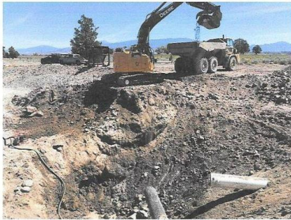
Below: Installation and backfill of water source pipes
