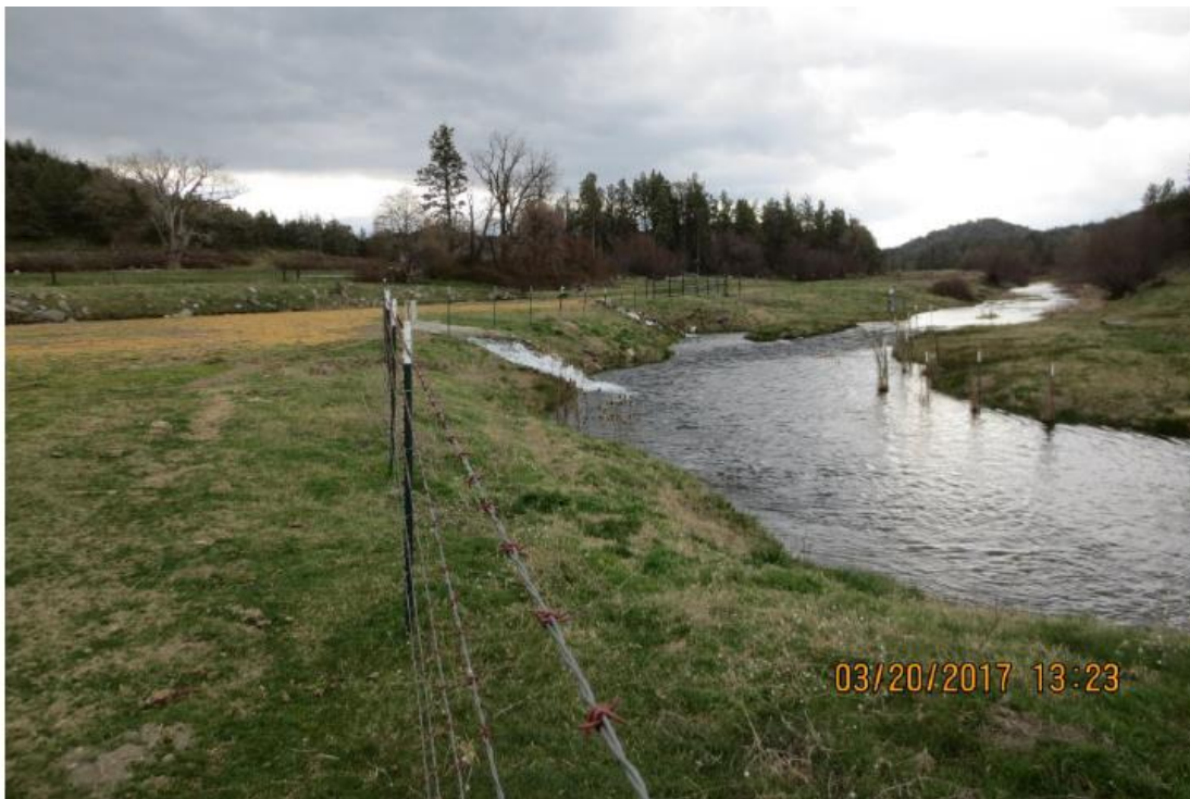
Post construction HV4D_PC_3.20.17
